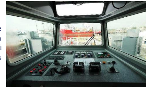
Aft bridge console with remote FiFi controls
