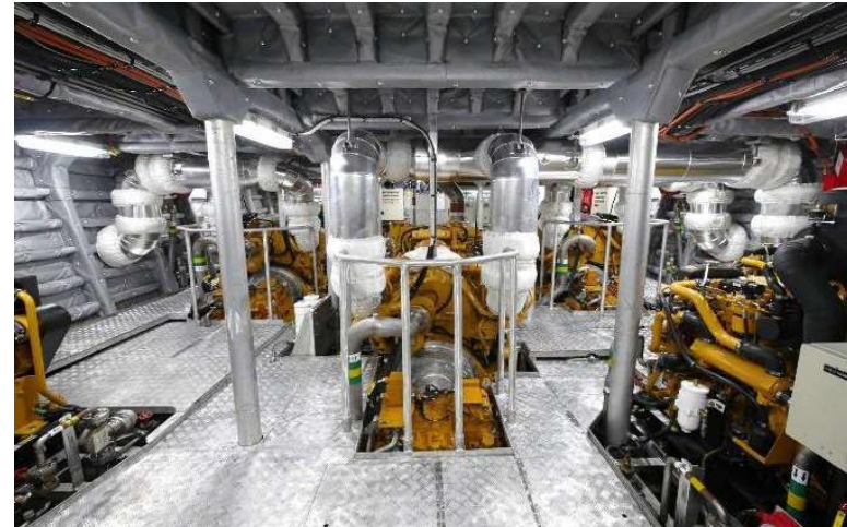
Spacious engine room
